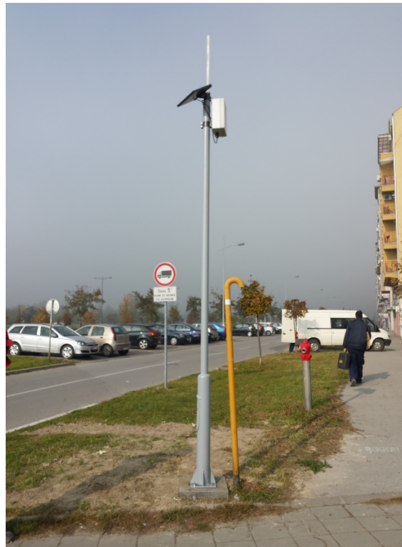
Fig. 6. TECHART Remote Monitoring Unit (TE-RMU) for buried pipelines
