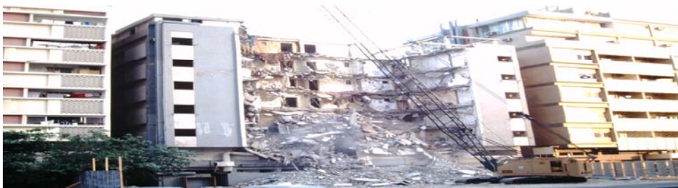
Fig. 1. Seventeen Year Old Building Being Demolished in Abu Dhabi due to Corrosion Damage
